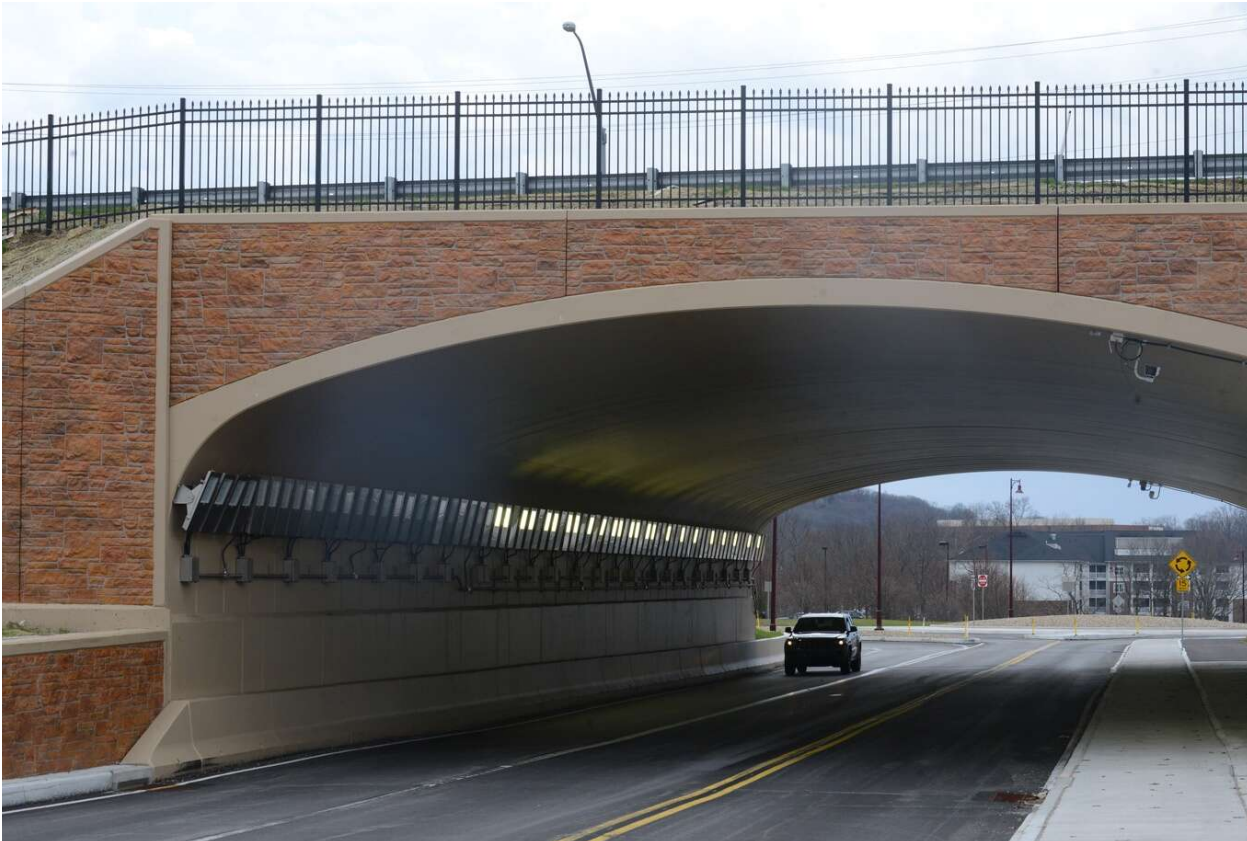
A car travels through the MSA Thruway tunnel in Cranberry Township. Julia Maruca/Butler Eagle
